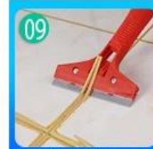
09 Don't touch in 4-5 hours and remove excess grout then.
