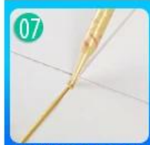
07 Evenly squeeze out the tile agent along the gap
