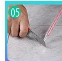
05 Inclined cut the top of the nozzle in 45°
